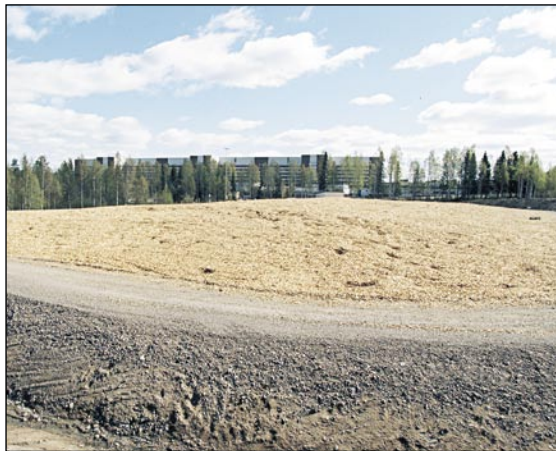
The snow reservoir is the size of a football pitch. In the spring the snow is covered with 20 cm of wood chips.
